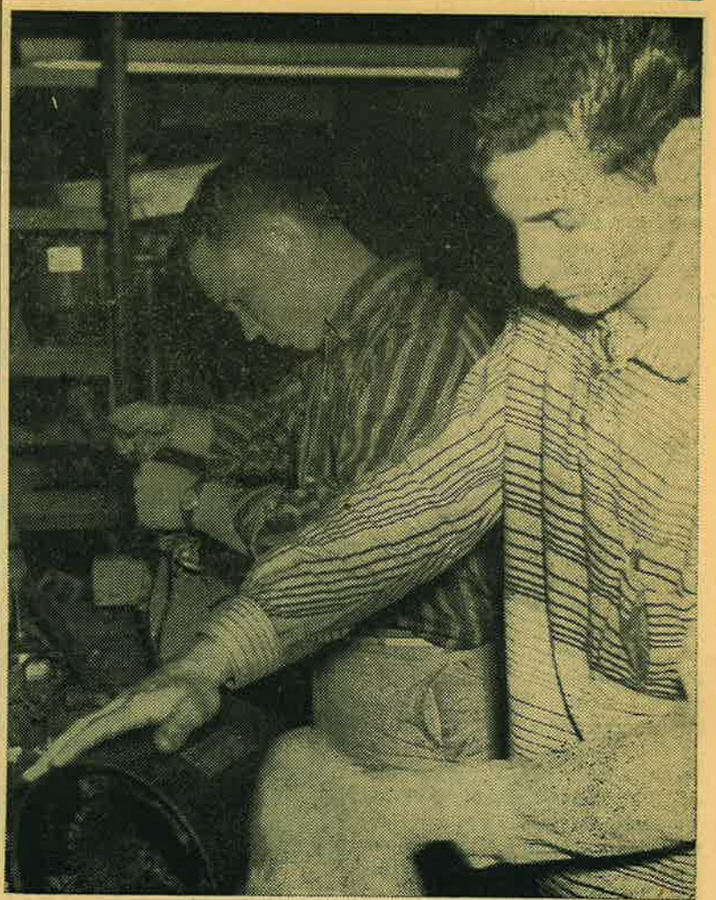
REWIND JOB—Conrad Lowery, front, and Merle Ehat are shown rewinding an electric motor in the Fresno Junior College electric shop. Cozy Photo
