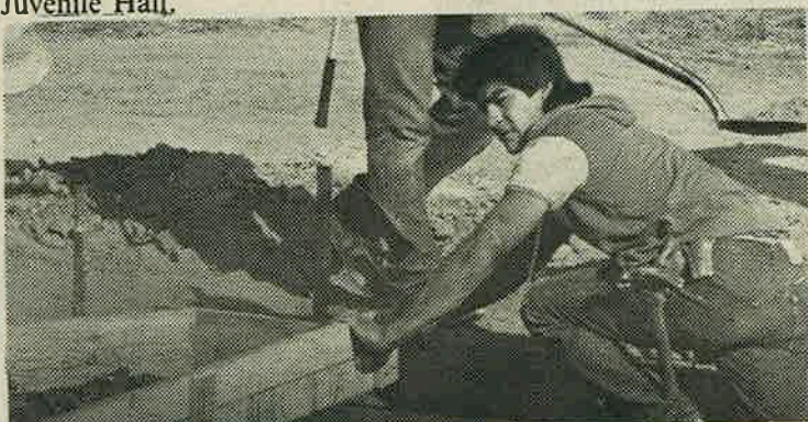
FCC construction students prepare for pouring of cement slab with the use of a wood slat bar. /Edward A. Garcia
