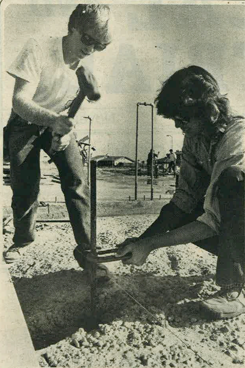
FCC students, Derek Smith (left) and Dominique Pardue (right), work together driving in iron post level guide during a construction class session.
