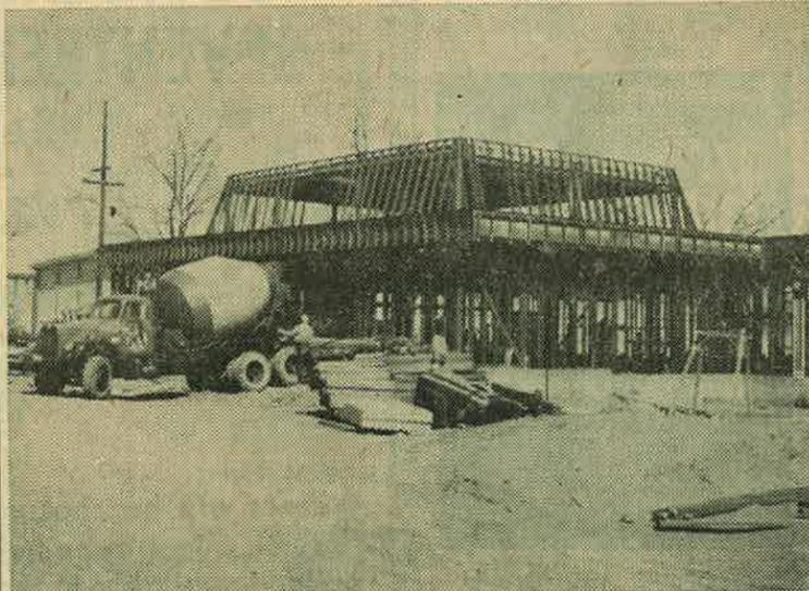
THE RIB STRUCTURE of the new cafeteria begins to take even more form as the architects begin to put the roof on the building. Planned for a fall completion, the cafeteria and coffee shop is designed to blend with the architecture of the recently completed gymnasium located across the street. The building will complete a mall from the University Ave. parking area with the gym entrance at the Weldon Ave. end. The present cafeteria will be remodeled into a student lounge and offices. (Clark Photo)
