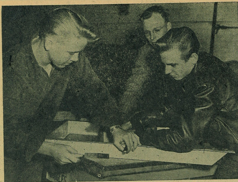
TWO SHEET METAL students rivet a louvre under the supervision of Frank Melton, instructor. The shop men are, left to right, Jimmy Baggett and August Koehler.
